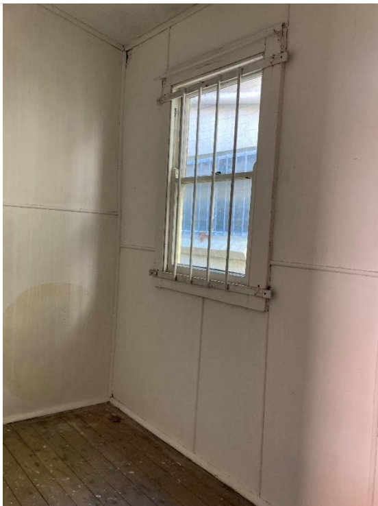
Figure 37: Timber framed single-hung windows with metal grill.
