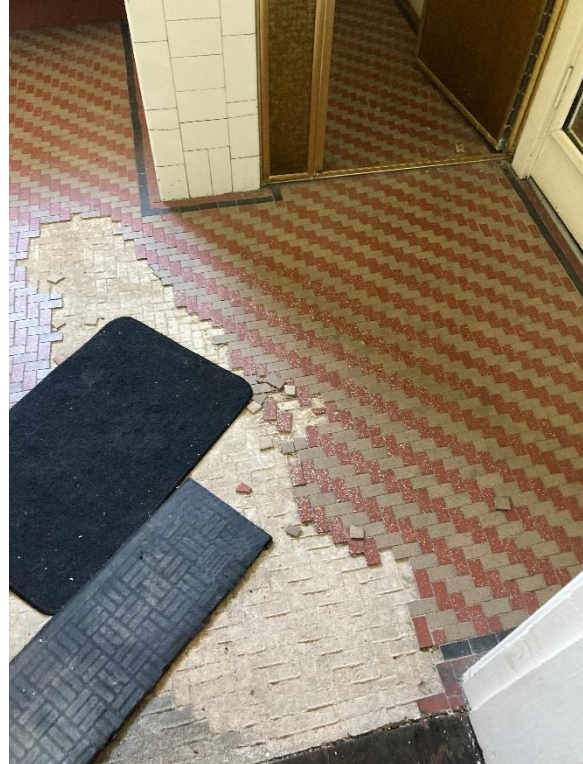
Figure 63: Damaged tessellated floor tiling at first floor toilet facility.
